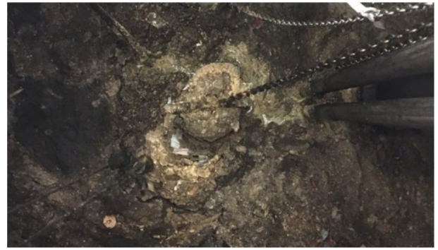
Figure 1. Lift station highly impacted by wastewater FOG loadings. Accumulated grease requires frequent removal and disposal.
